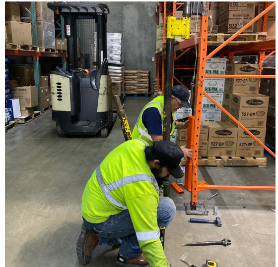
STEP #2 - SUPPORT DAMAGED UPRIGHT
